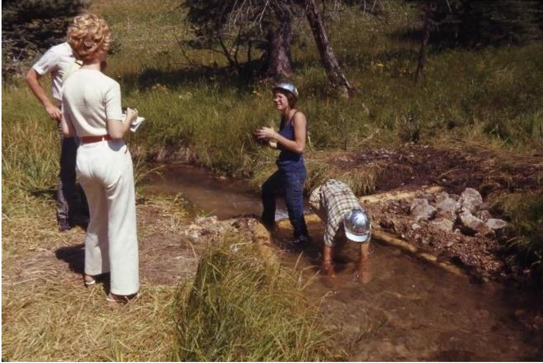
Figure 86. Construction of a weir from logs and rocks on a creek, Youth Conservation Corps, Camp Judson, 1970-79. Courtesy of Black Hills National Forest Historical Collection, Leland D. Case Library for Western Historical Studies, BHSU (Identifier BHN20160501).
