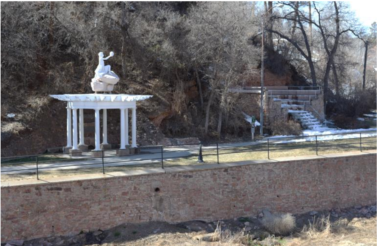
Figure 81. A stone retaining wall along Fall River in the Hot Springs Historic District. Photo from SD SHPO.
