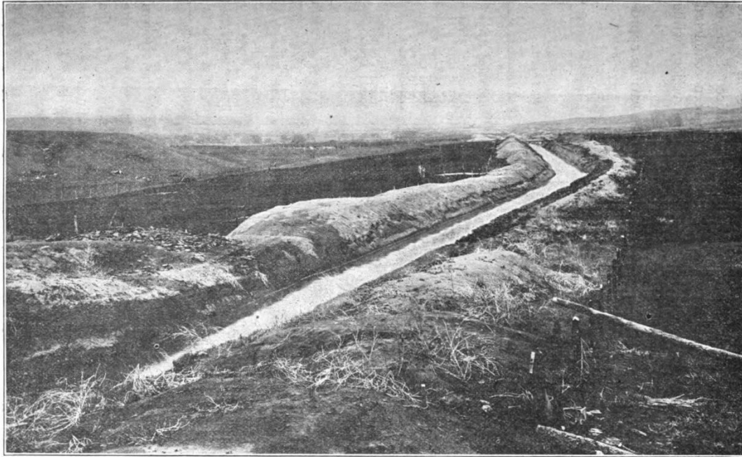
Figure 27. Canal to the Black Hills Traction Company's hydroelectric plant.
