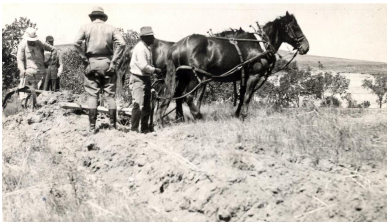
Figure 55. CCC-ID workers digging lateral at Soldier Creek on the Rosebud Indian Reservation (Rosebud Sioux Tribe). Courtesy of the National Archives (Identifier 12080193).
