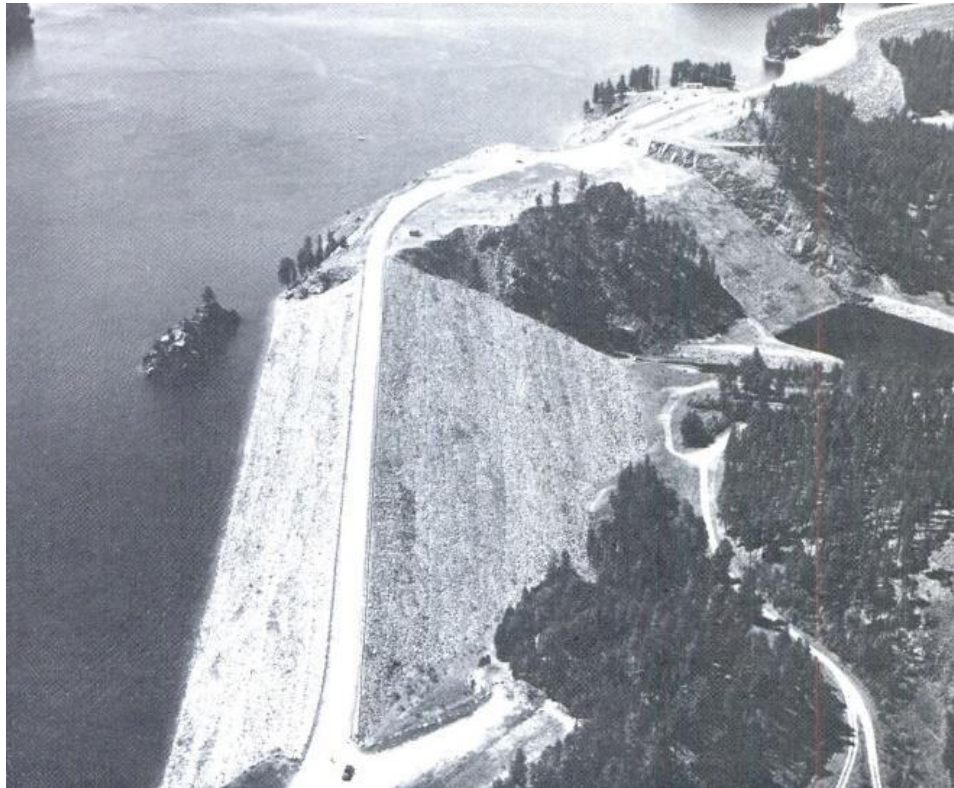
Figure 60. Pactola Dam and Reservoir. Courtesy of the Bureau of Reclamation.
