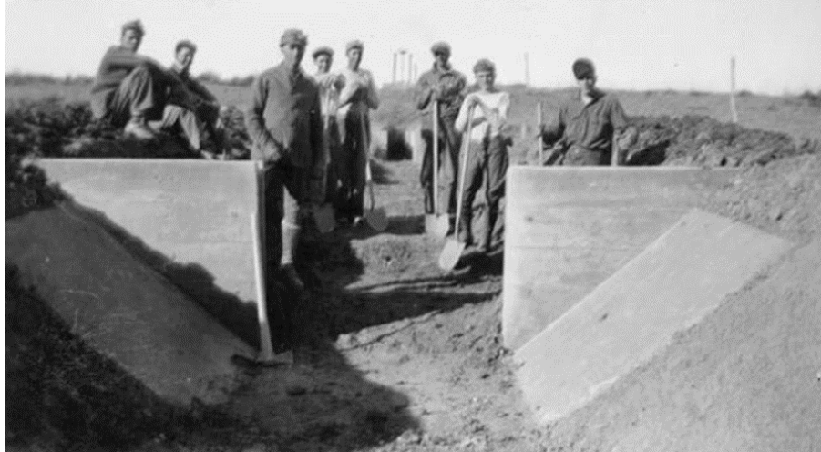
Figure 49. CCs working on the Belle Fourche Dam. An inscription indicates this photo was taken after a canal gate was built at the end of a siphon and shows enrollees standing near a finished gate and ditch cleared out by the crew. Courtesy of the SDSHS, South Dakota Digital Archives (2010-08-31-018).
