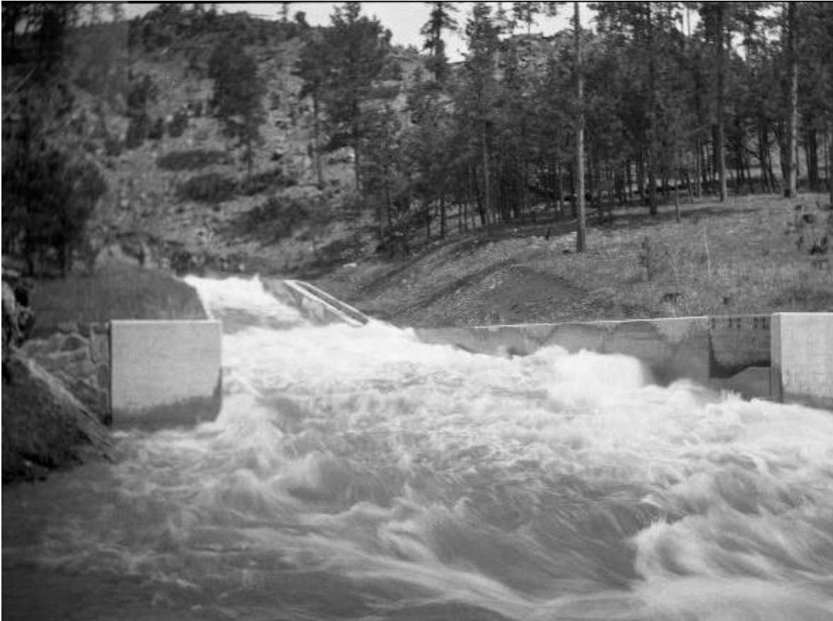
Figure 85. Lower end of stilling basin of Sheridan Dam and Dakota Lake, where run-off water enters Spring Creek channel. Fish ladder and fish ladder well on right side. Courtesy of Black Hills National Forest Historical Collection, Leland D. Case Library for Western Historical Studies, BHSU (Identifier BHNF20151576).
