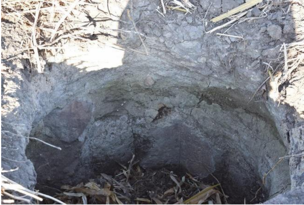
Figure 76. Well lined with brick, mortar, and stone at Site 39HT0147. 454
