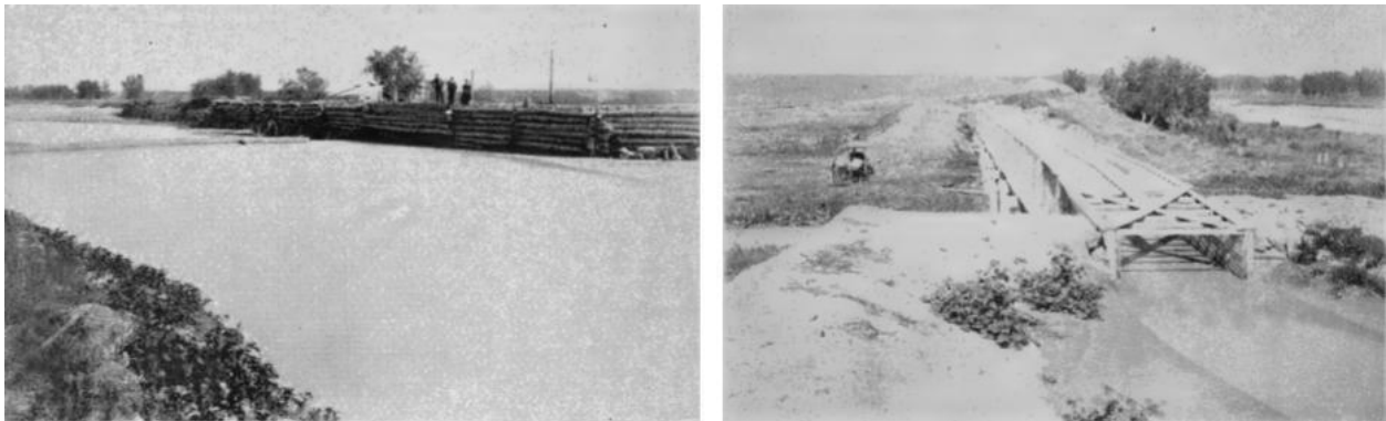
Figure 7. "Dam and headgate in Cheyenne River at head of the Edgemont Canal" (left); "Flume carrying canal water over Moss Agate Creek" (right).
