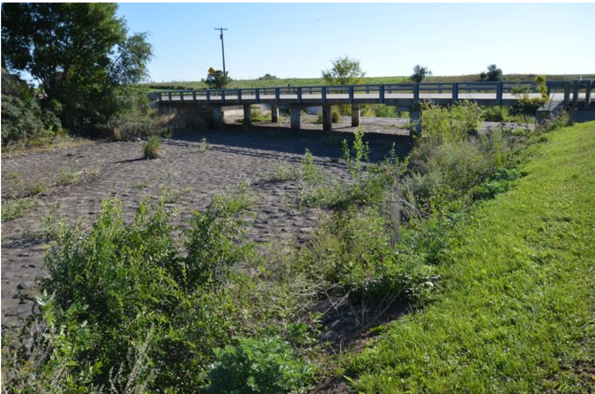
Figure 94. This 1999 bridge crosses the top of the stone-lined Richmond Lake Dam, northeast of Aberdeen. Photo by SD SHPO.
