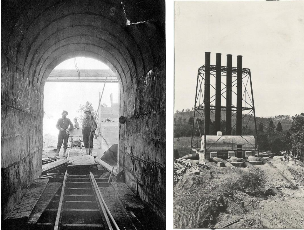
Figure 32. LEFT: Teams standing at the entrance of a tunnel under construction. Approximate length of tunnel 24,000 feet, approximate dimensions 6'6" wide by 9' high. Courtesy of Deadwood History, Inc. (Identifier 13-2). RIGHT: Four standpipes at Hydro No. 1. Courtesy of Deadwood History, Inc. (Identifier 10-5).
