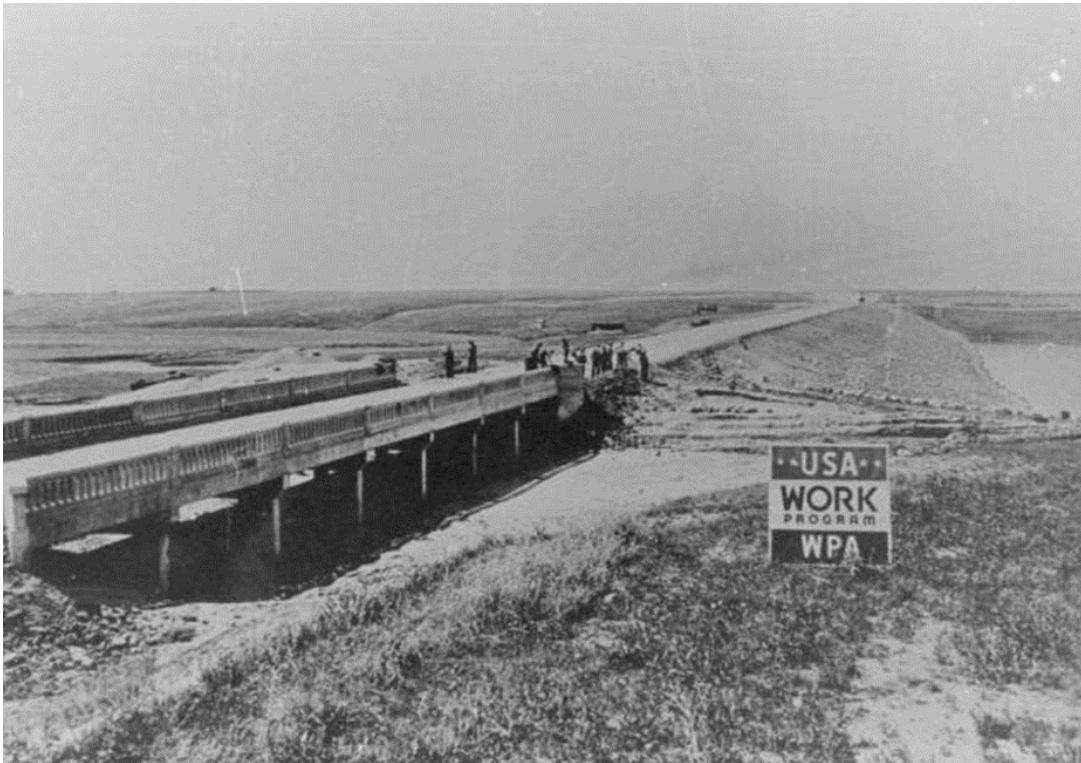
Figure 41. Drought-stricken farmers working on a dam to mitigate the impacts of future droughts in Aberdeen, Brown County, South Dakota. Note the “USA Work Program WPA” sign in the foreground. Courtesy of the SDSHS, South Dakota Digital Archives (2017-08-07-318).
