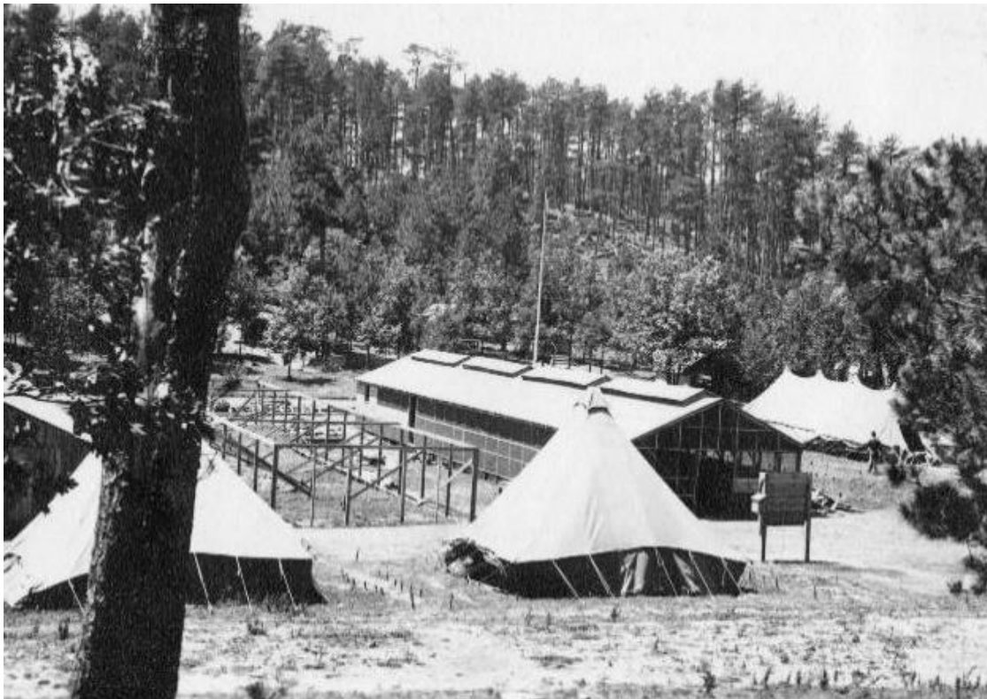
Figure 96. Row of barracks buildings (20' x 80') being constructed at the Rockerville CCC Camp F-10, Company 1794. Courtesy of Black Hills National Forest Historical Collection, Leland D. Case Library for Western Historical Studies, BHSU (Identifier BHNH20221642).
