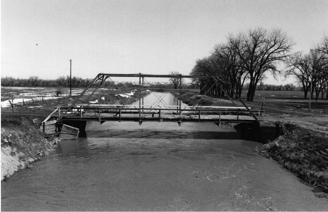
Figure 93. Bridge 10-109-360, Butte County, South Dakota. Photograph from National Register nomination.
