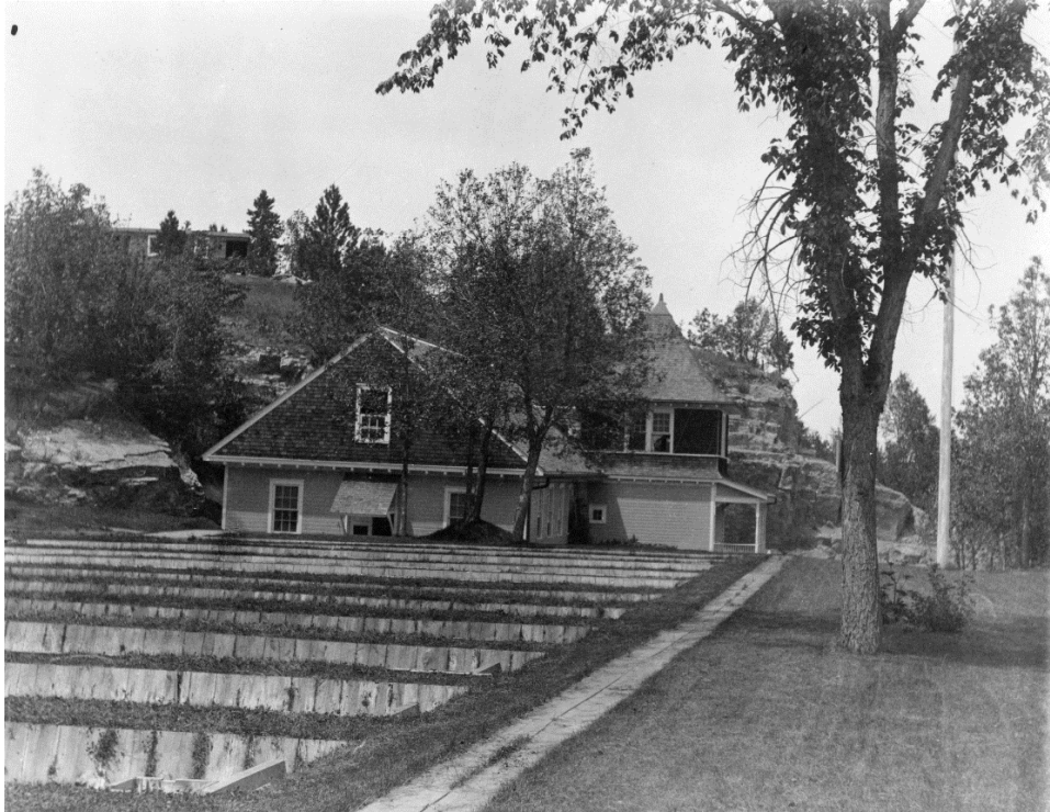
Figure 37. An undated photograph of Spearfish National Fish Hatchery, now known as the D. C. Booth Historic National Fish Hatchery, in Lawrence County. The coupled raceways shown in the foreground were built by the WPA in the mid-1930s. Courtesy of the Cook Photograph Collection, Leland D. Case Library for Western Historical Studies, BHSU (Cook20220038).
