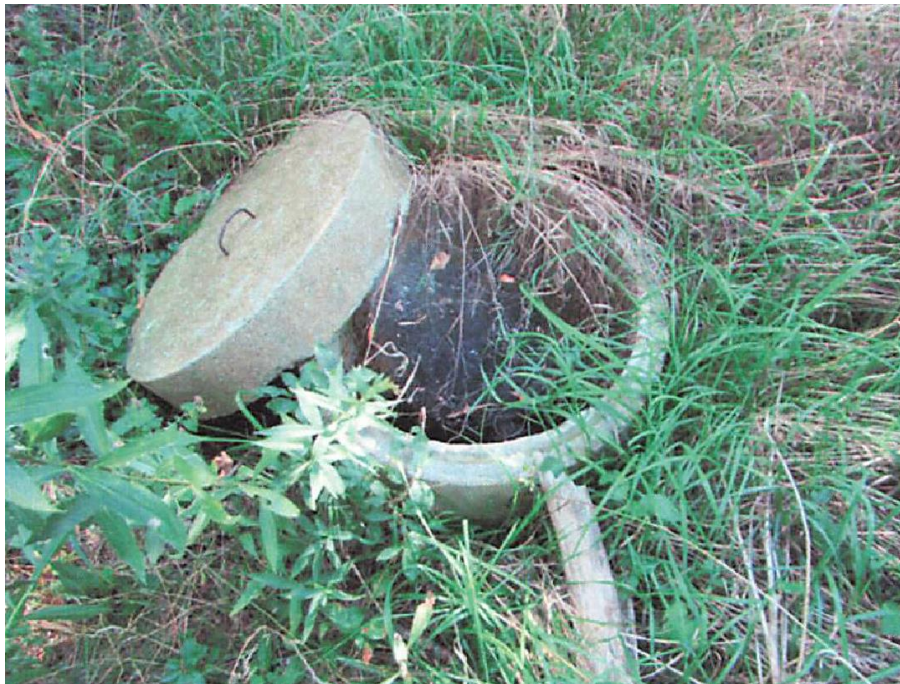
Figure 75. Concrete cistern recorded at Site 39MH332, Minnehaha County, SD. 453
