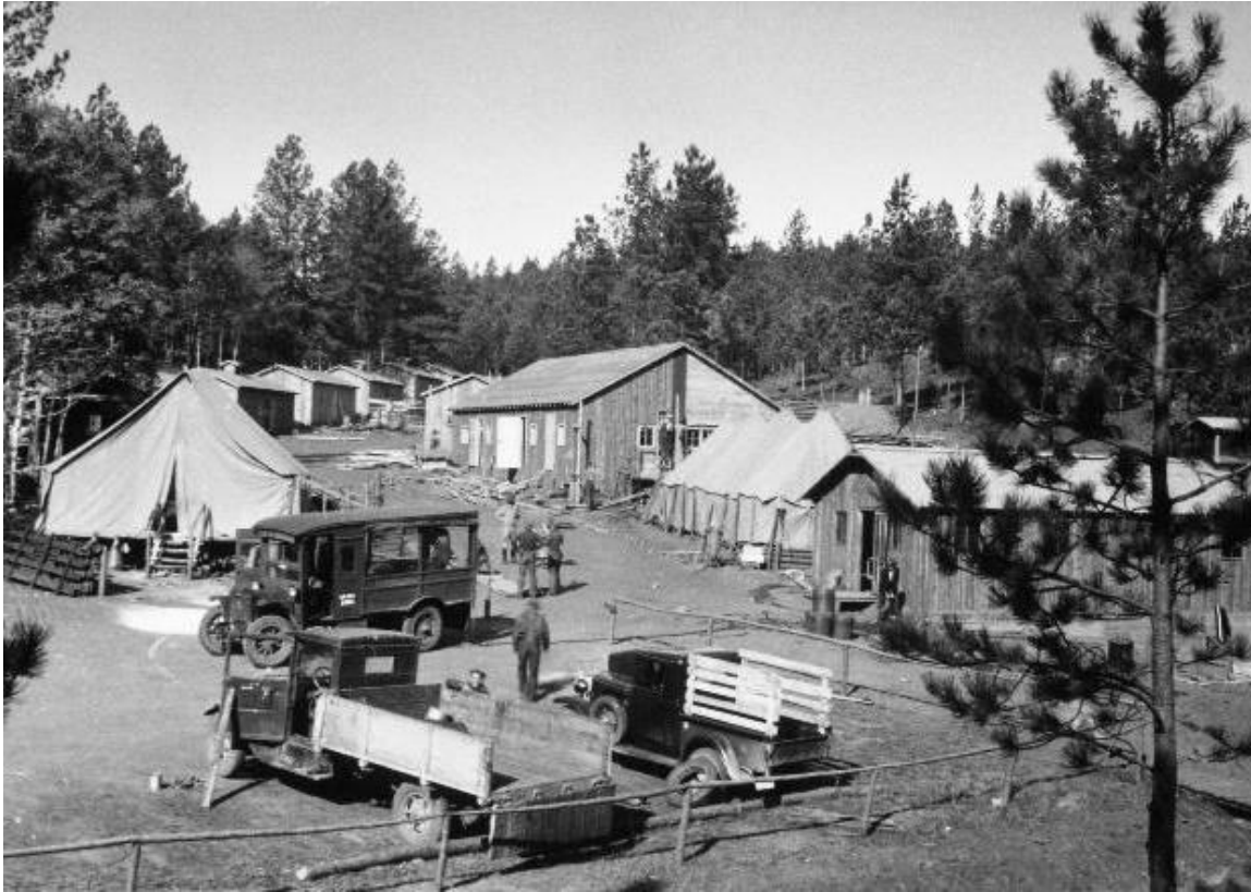
Figure 97. Buildings in the process of construction at Rochford Camp F-5, showing Company Street with mess hall in right foreground. Courtesy of Black Hills National Forest Historical Collection, Leland D. Case Library for Western Historical Studies, BHSU (Identifier BHNH20210251).
