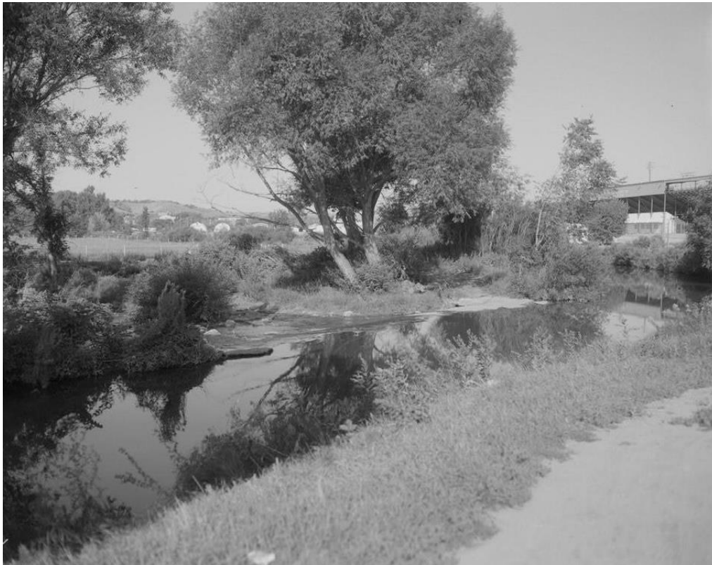
Figure 4. The diversion dam and intake canal of the Hawthorne Ditch as it looked c. 1995. The diversion dam, made of boulders with concrete facing, was built across Rapid Creek and channels water to an intake canal. The diversion dam and intake canal are some of the only remaining examples of historic headworks in farmer-owned irrigation ditches in the Lower Rapid Valley. Courtesy of the HAER (SD,52-RACI.V,2).
