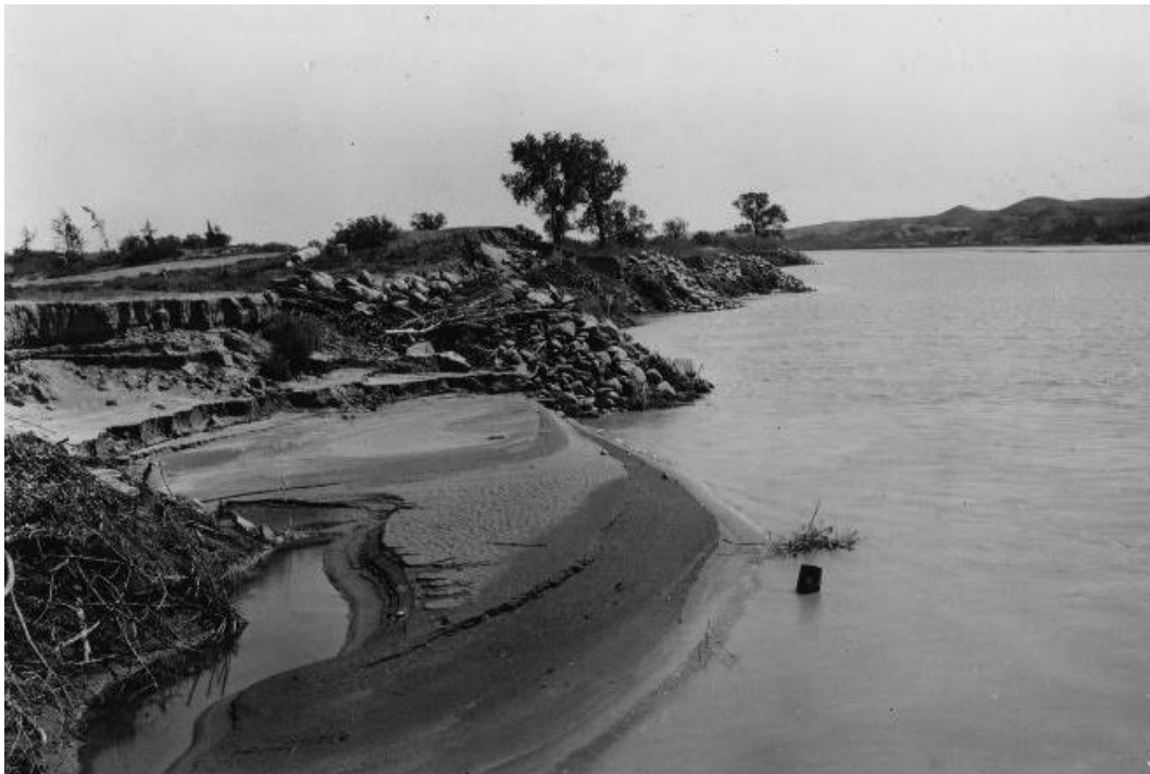
Figure 77. Rock jetties on south side of Farm Island to protect the south shoreline (work completed by CCC enrollees). Courtesy of Black Hills National Forest Historical Collection, Leland D. Case Library for Western Historical Studies, BHSU (Identifier BHNF20144654).
