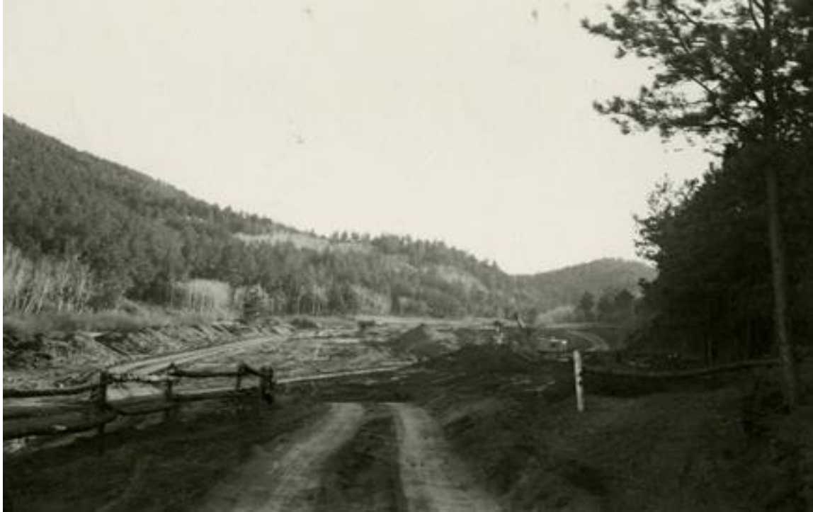
Figure 98. Mallory Gulch borrow pit at Sheridan Dam, taken in 1939. Courtesy of Black Hills National Forest Historical Collection, Leland D. Case Library for Western Historical Studies, BHSU (Identifier BHN20151512).
