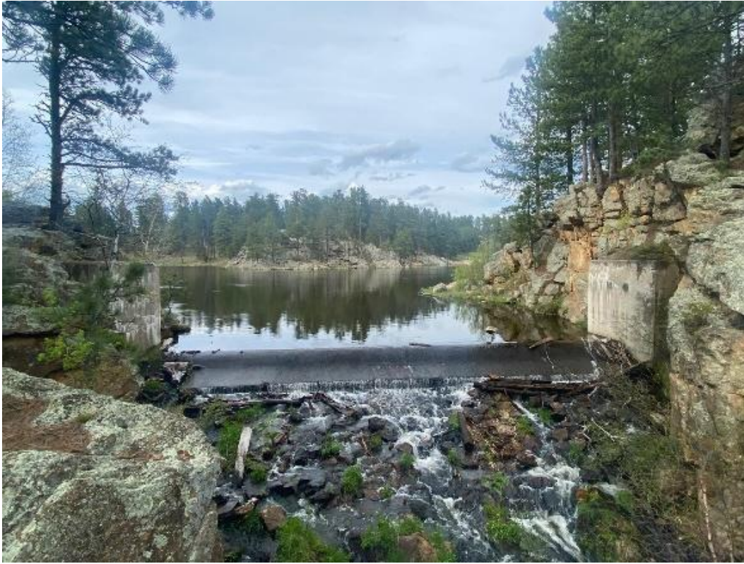
Figure 82. Bismarck Lake Dam, taken in 2024.
