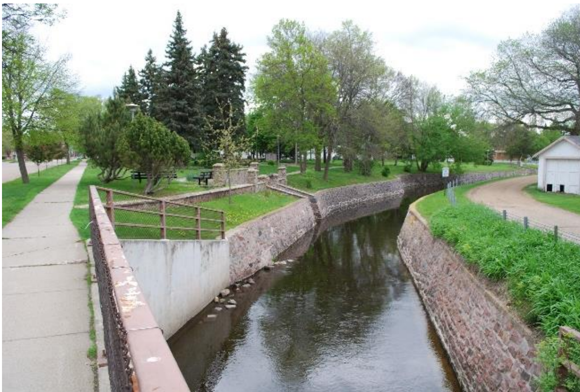
Figure 71. Madison City Canal at Memorial Park in Madison, SD. Courtesy of SD SHPO.
