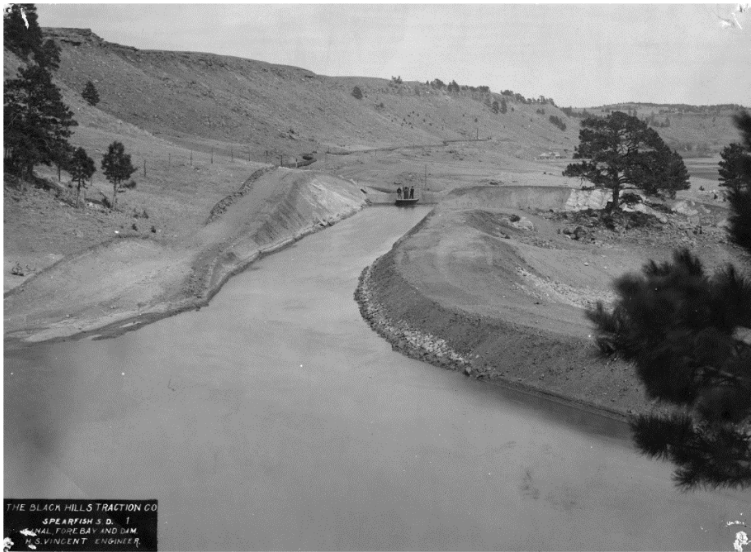
Figure 28. A photograph of the canal, forebay, and dam of the Black Hills Traction Company. Courtesy of the Leland D. Case Library for Western Historical Studies, Black Hills State University (BHSU) (Identifier BHA20220003).
